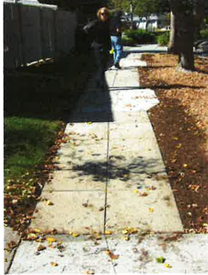
Rubber Panel Installation
