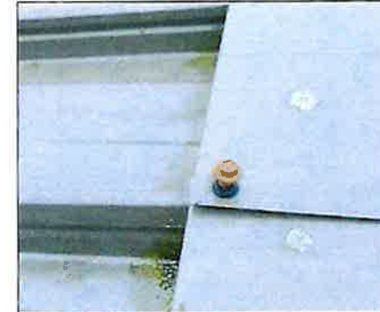
Replace all backing out fasteners.
