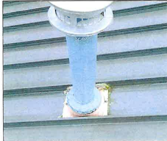
Replace all pipe boots set in sealant.
