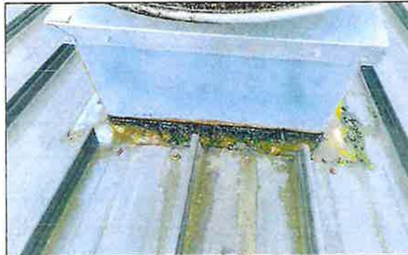
Prep, Prime and Paint rusting areas around penetrations.
