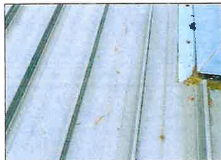
Prep, Prime and paint areas where coating is peeling away.
