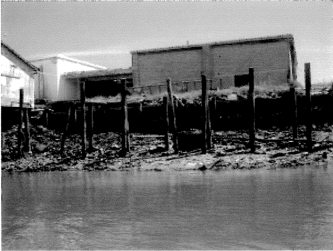
Photo 3. Failing bulkhead near center of Project area.
