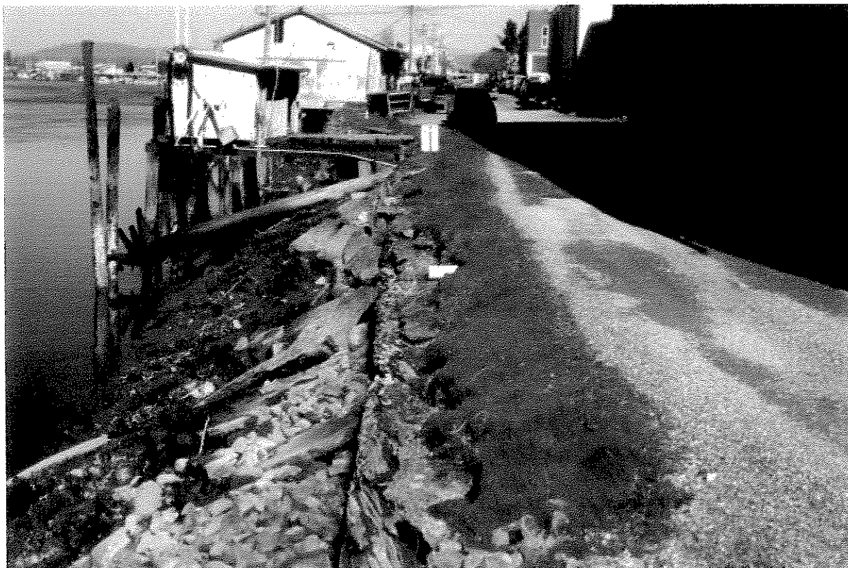
Photo 2. View of Project area from southern boundary showing failing bulkhead and concrete slab riprap.
